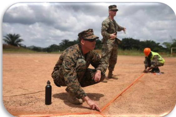
U.S. Marines and Liberian troops set up a landing zone at the construction site of an Ebola treatment center on October 11 th in Tubmanburg, Liberia. (John Moore/Getty Images)
